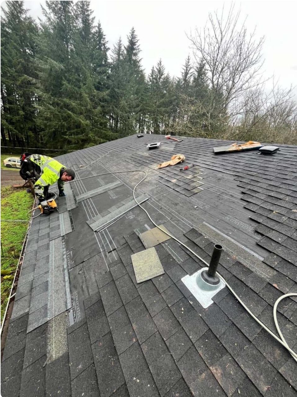
Architectural shingles being installed, showing their layered dimensional profile
