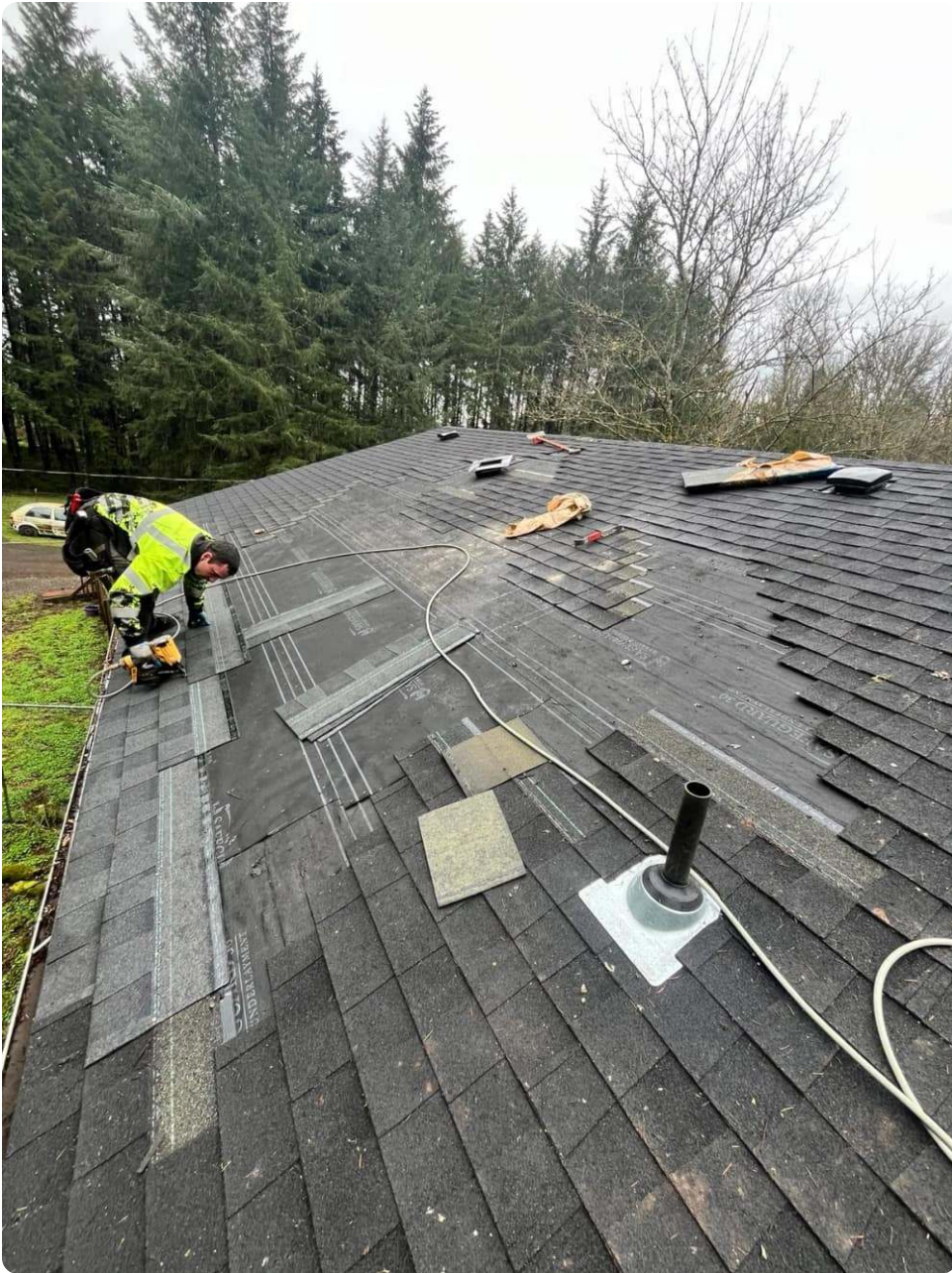
New architectural shingles being installed on a Damascus area home
