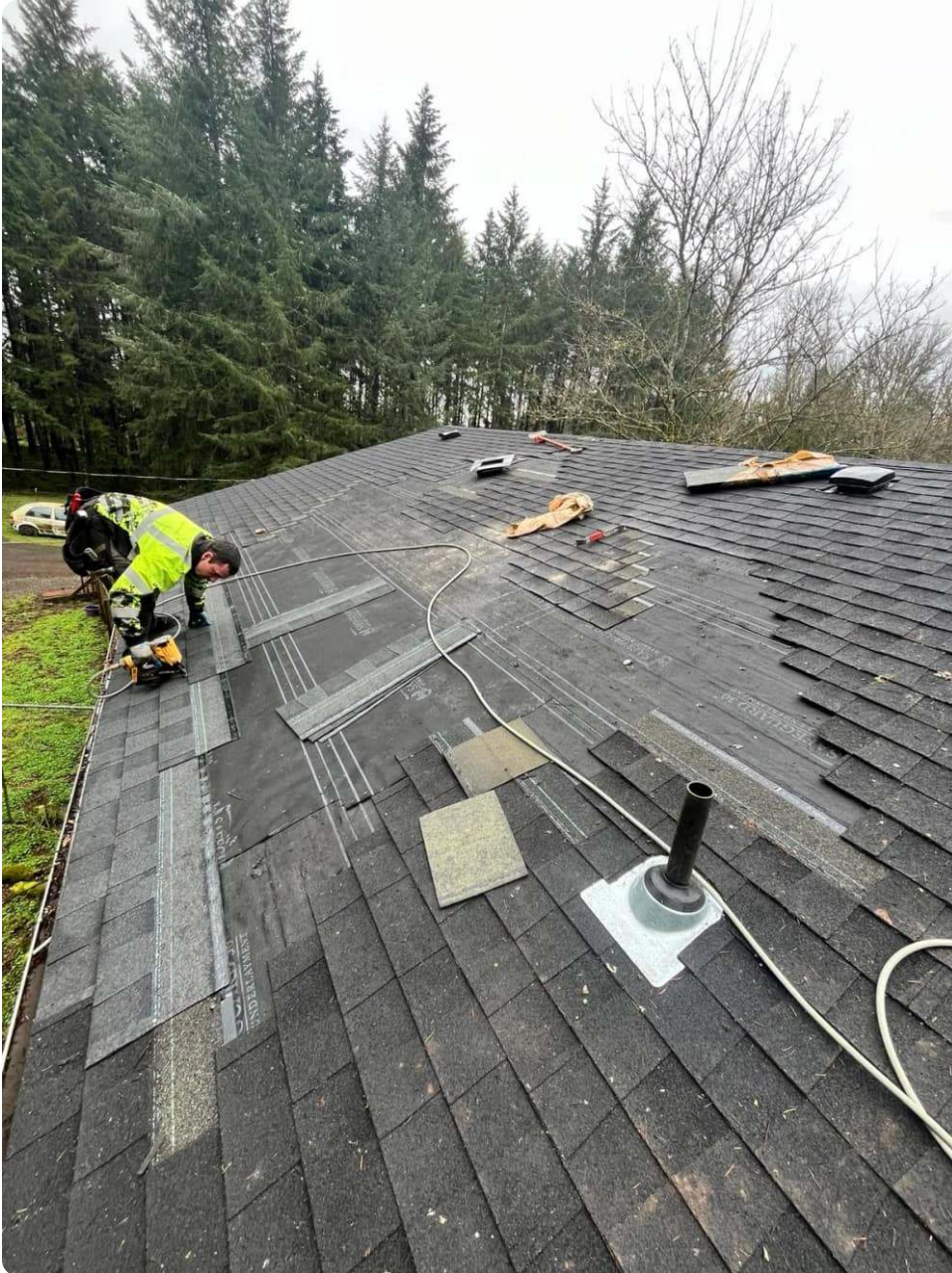
Architectural shingles being installed over underlayment
