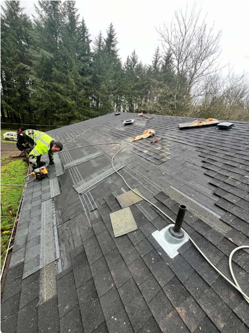
CertainTeed architectural shingles being installed by a certified crew
