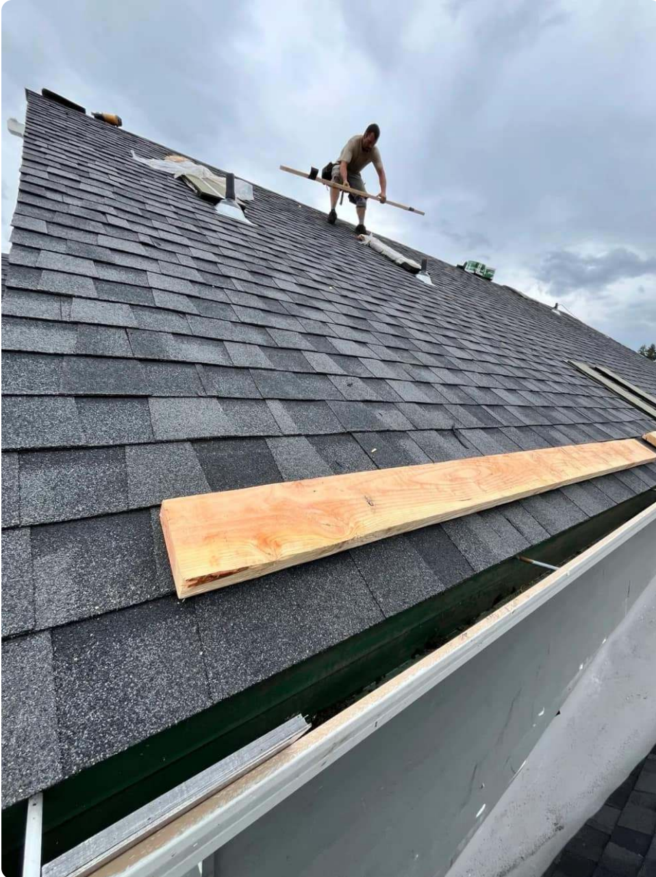
French Roofing crew member working along a roof ridge
