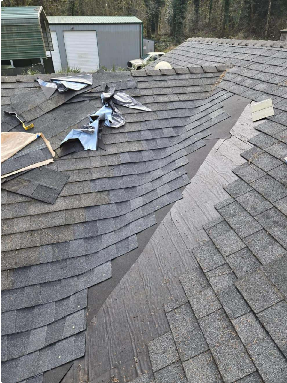
A roof valley being installed during a replacement
