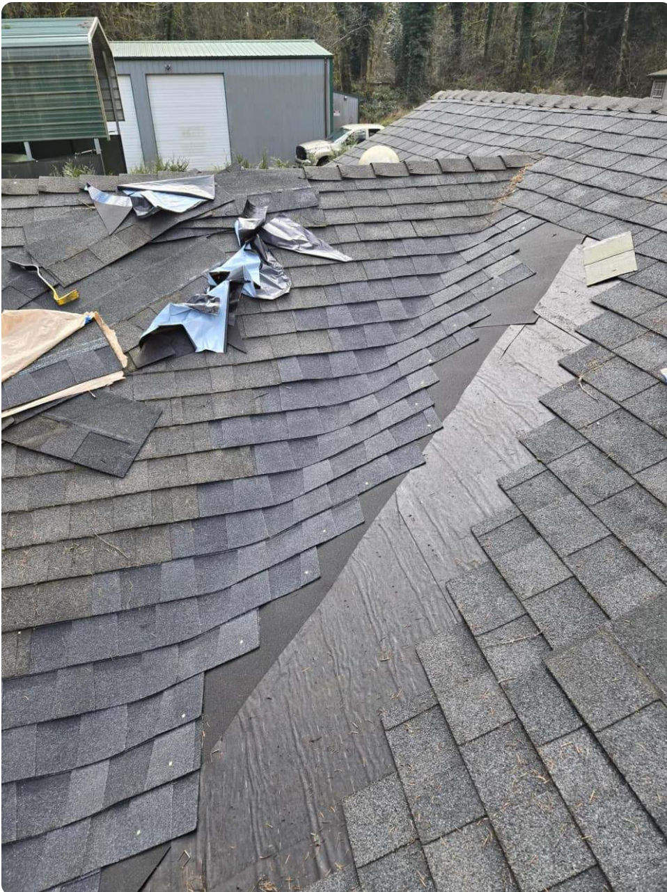
An open valley being installed with shingles trimmed to the channel
