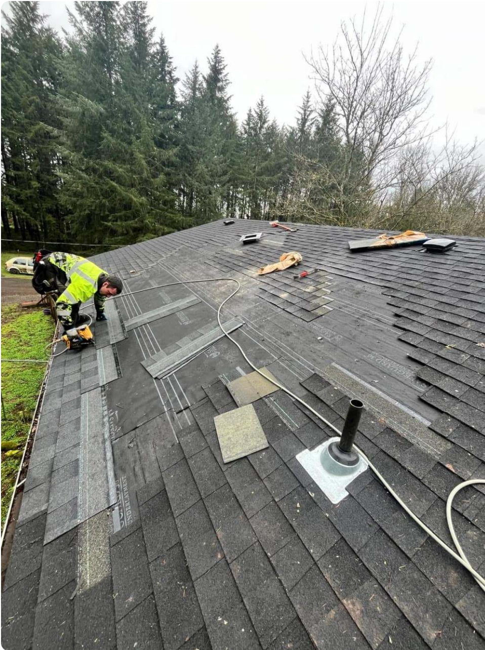
Architectural shingles from the mainstream product tier being installed
